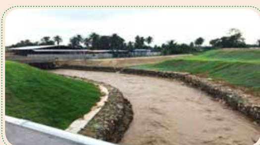
Banks are protected to ensure watercourse at Plot C06, Hemaraj CIE II
