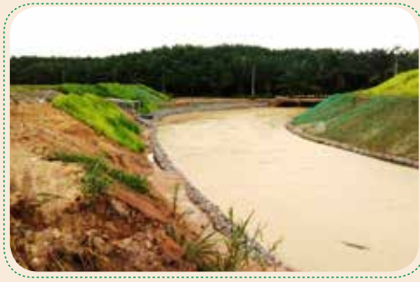
Canal banks are protected between Phase 3 and Phase 5 at Hemaraj ESIE
