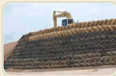
Steep Slope Reinforcement using soil bag reinforcement and Geogrids facing Plot A11B, Hemaraj RIL.
