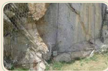
Slope Protection with rockfall netting at Plot PX31 (MAZDA), Hemaraj ESIE
